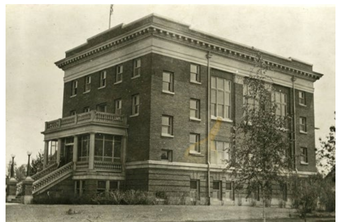
View of the Charles Thompson Memorial Hall building on November 11, 1916. The building was designed by the architect Olof Hanson, who was deaf.
